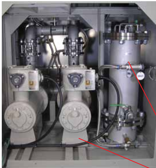
Water Conditioning System
