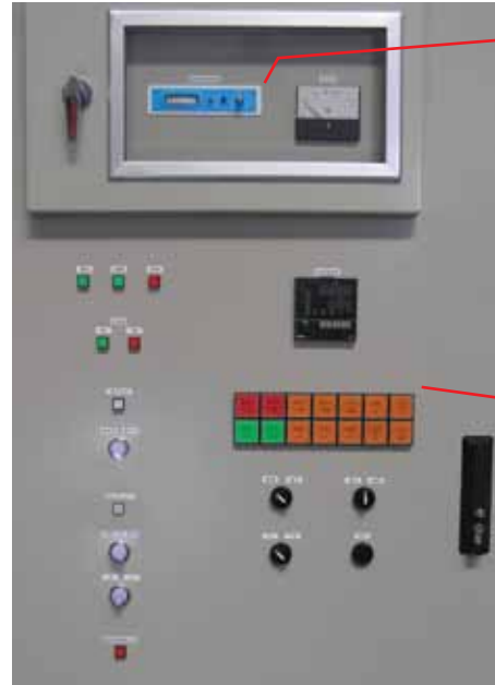
Interface and Water Cooling Panel
