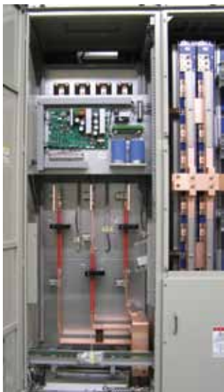
Rear of Interface Panel – Motor Connections at Bottom
