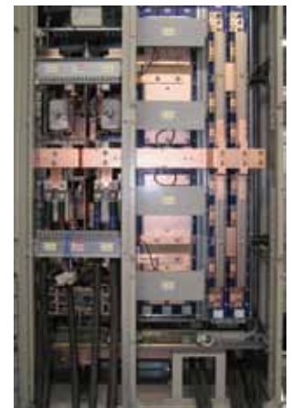
Rear of U-Phase
