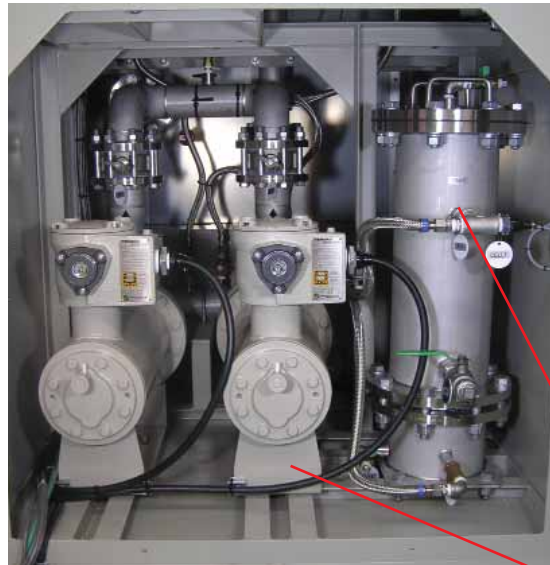
Water conditioning system behind Gate Drive Panel
