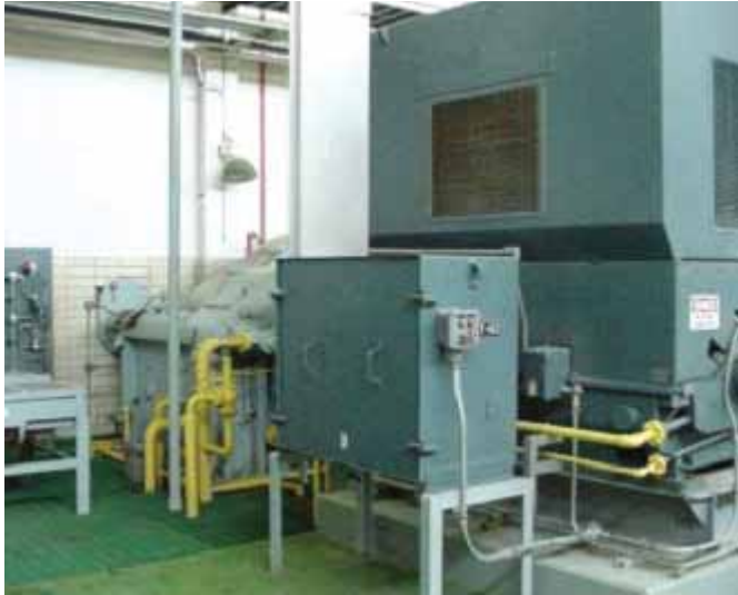
Induction Motor and Gearbox (compressor located on the other side of wall)
