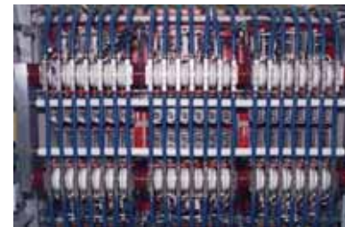
One channel power bridge showing thyristor (SCR) stacks and water cooling.
