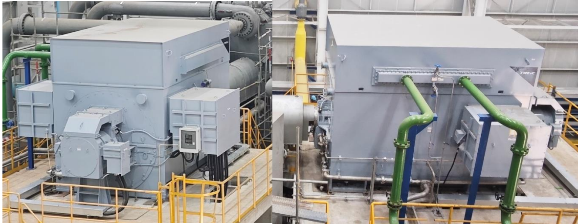
6-pole large synchronous motor developed by TMEiC (Output: 48.4 MW)
