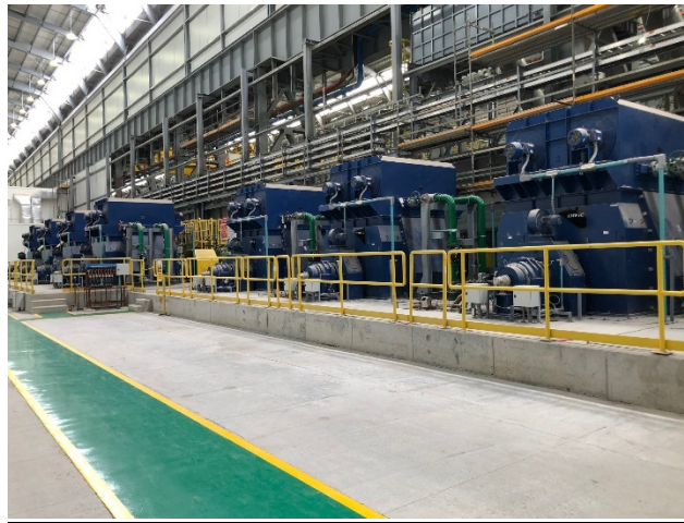
Motors delivered by TMEiC
