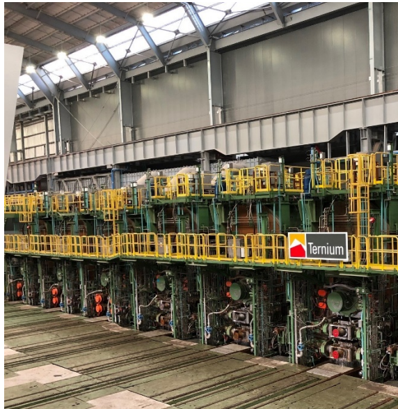
Newly established hot strip mill
