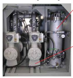
De-ionizer removes contaminants from the internal cooling loop.
