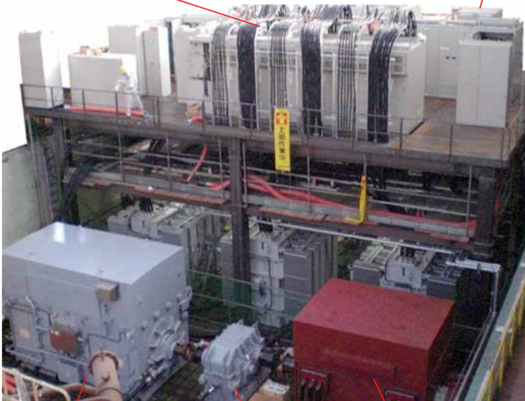
Regenerative TMdrive-70 three-level IEGT drive to recirculate power back to the supply
