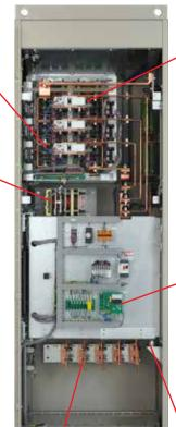
Main Power module. One module is applied for the 1200A supply and two modules for the 2100A model.
