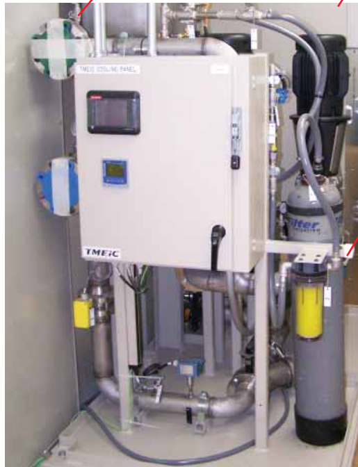
Water conditioning system behind Gate Drive Panel
