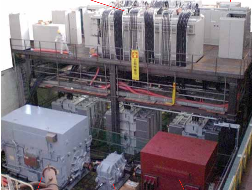
Regenerative TMdrive-70 three-level IEGT drive to recirculate power back to the supply
