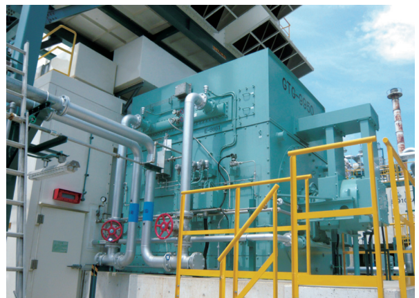
4-Pole Synchronous Generator 4P-37MVA, 11kV 60Hz Ex-p | Oil Refinery
