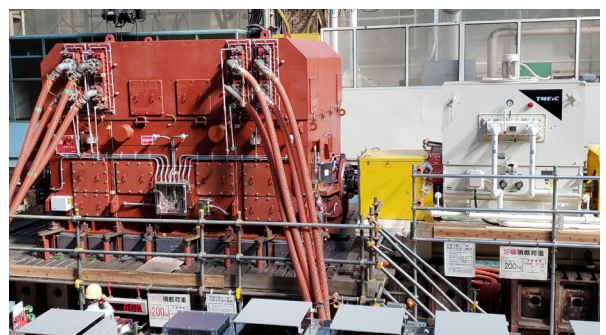
2019 || TMEIC 2-Pole, 40MVA, Water cooled Turbine Generator designed with matched dimensions to replace existing unit
