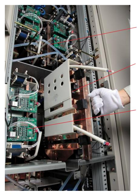
Flexible Water Cooling Tubes are easy to manage when performing maintenance.
