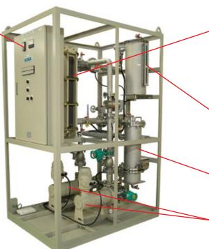
Water to water heat exchanger keeps the de-ionized system isolated from the plant water supply.
