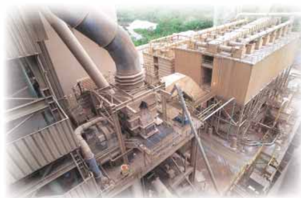
Induced Draft (ID) Fan In Cement Plant
