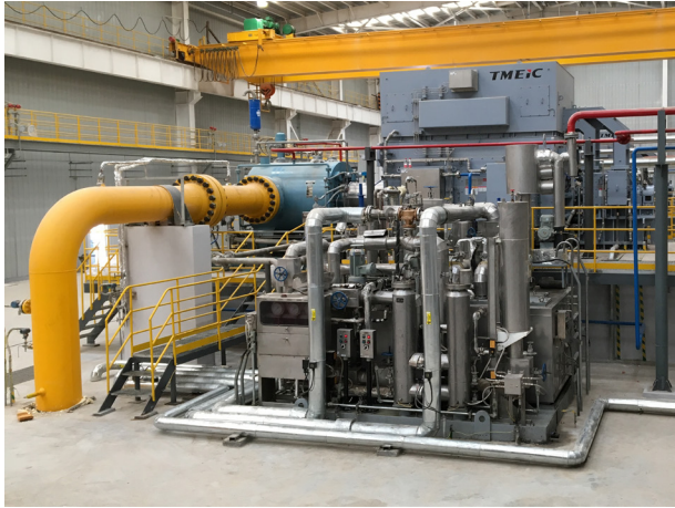
Figure 1. High speed direct-drive motor-compressor (18 MW, 5460 RPM).
