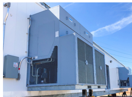
Image 3. VFD E-house showing substantial HVAC units
