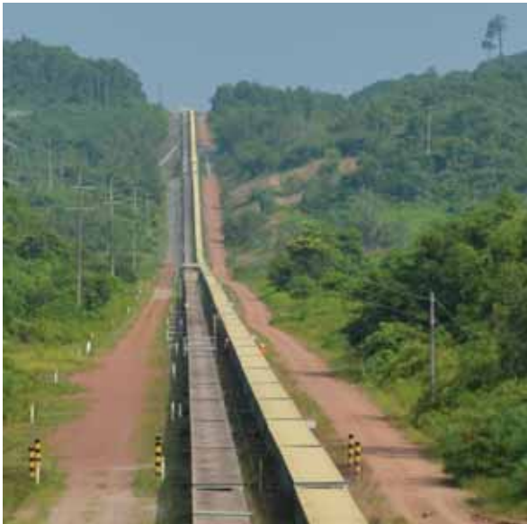
Typical overland conveyor
