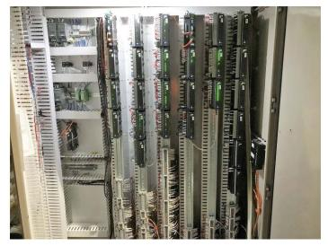
Figure 20, new nV Remote I/O
