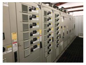
Figure 14, New Furnace Drives
