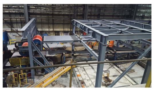
Figure 5, New Steel Super Structure to support Furnace Extension
