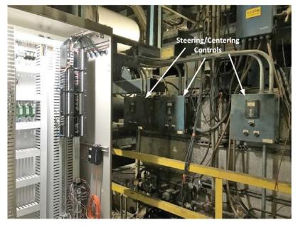
Figure 10, Steering/Centering Controllers (indicated by arrows) were replaced with new remote I/O (left) and nV Controllers
