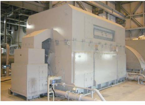
For IPP 2-pole Air-cooled Turbine Generator In Water-cooled TEWAC Enclosure
