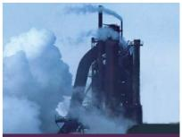
Generating power utilizing the surplus gas at steelworks to drive equipment such as top pressure recovery turbine (TRT) and coke dry-quenching (CDQ) co-generation systems, we're contributing to energy-saving environmental management.
