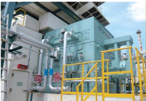
For IPP 4-pole Air-cooled Turbine Generator In Water-cooled TEWAC Enclosure
